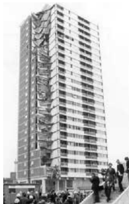
Ronan Point building after the May 1968 collapse.
